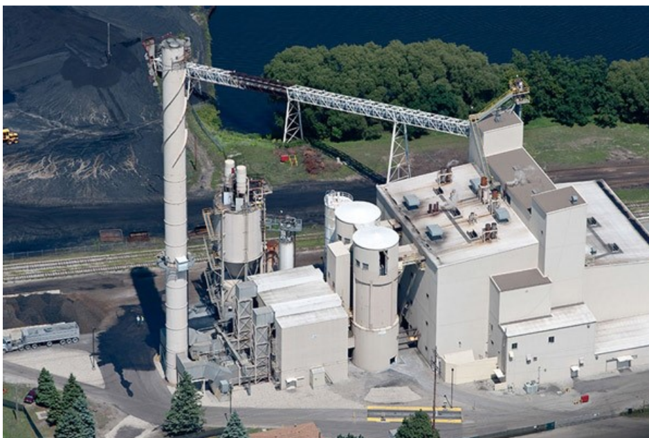
T.E.S. Filer City Station cogeneration facility | Tondur
