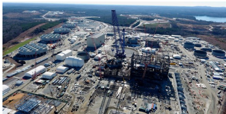
V.C. Summer expansion project | SCANA
